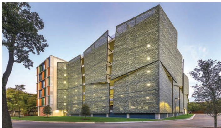
RICE UNIVERSITY – CAMBRIDGE OFFICE BUILDING Houston, Texas
